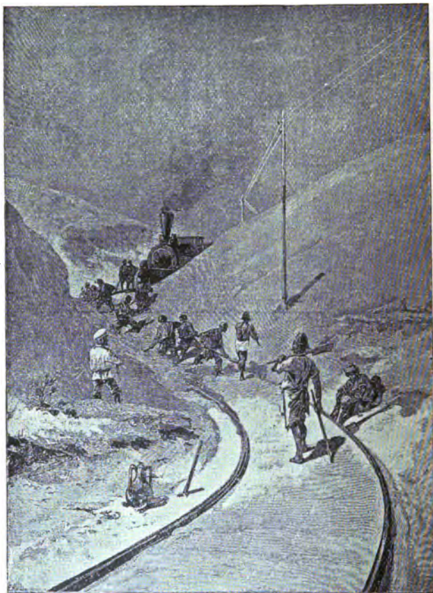
SWEEPING SAND FROM THE RAILWAY.
